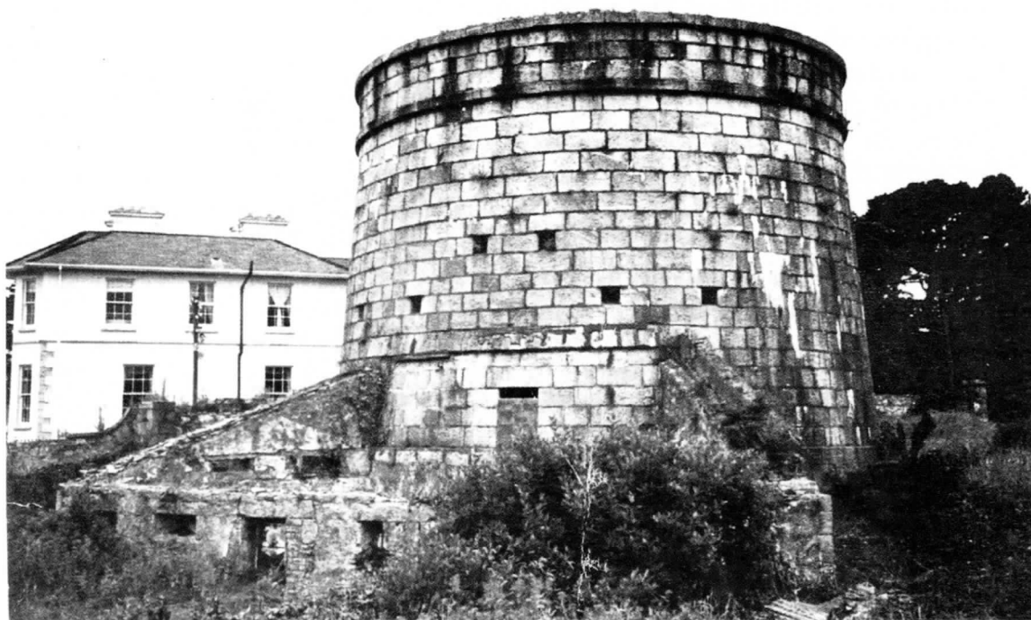
3. Tower Before Restoration 2 – viewed from the south-east/battery plain
